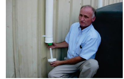
11 Check first flush collector
