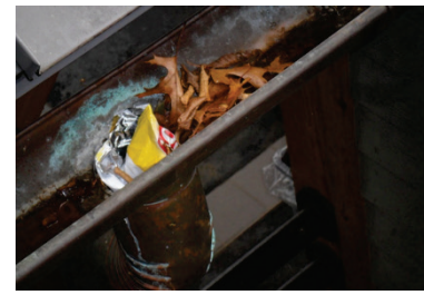
5 Clear gutter debris
