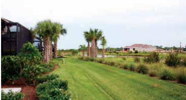
Swales encourage stormwater to soak into the ground.
