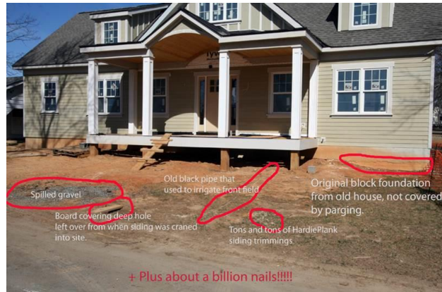
Typical soil at new home construction site
