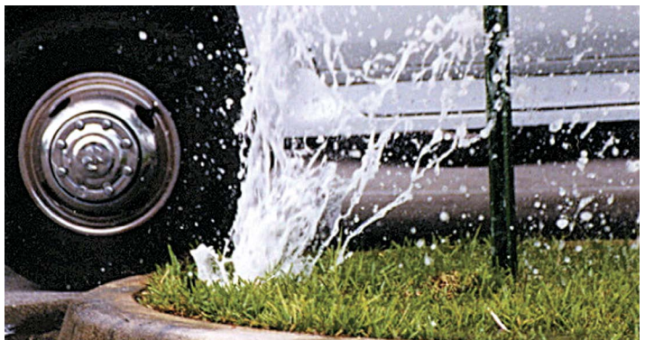
Figure 16. Water gushing from broken head.
