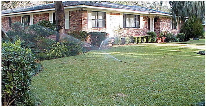
Figure 13. Poor design; system does not match irrigation requirements. The area needs to be rezoned with landscape and turf separated.
