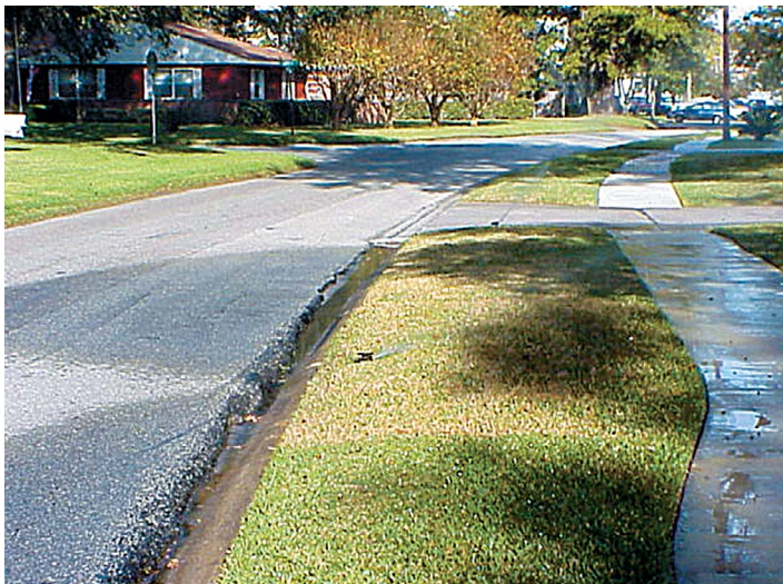
Figure 12. Poor design; sprinkler does not match area.
