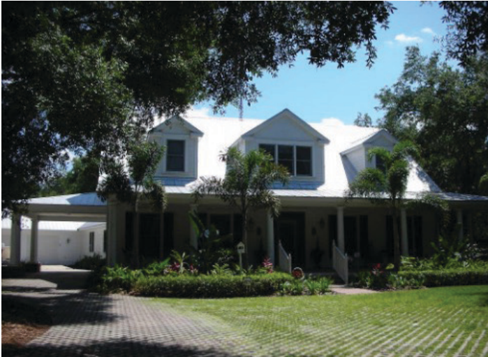
Figure 27. Pervious pavement. Credit: UF/IFAS Florida-Friendly Landscaping™ Program
