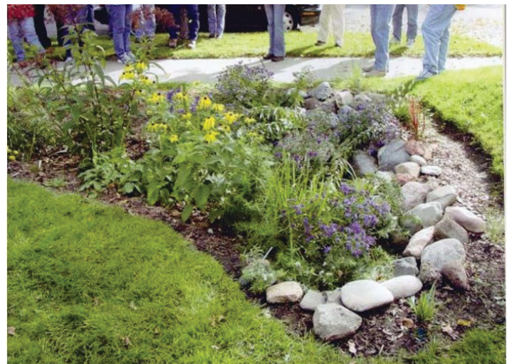
Figure 26. Rain garden. Credit: UF/IFAS
